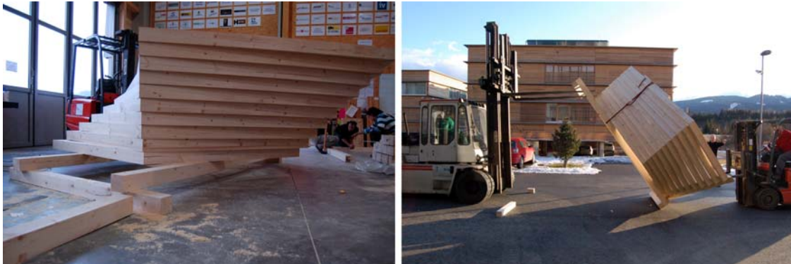
Figure 10 Combined transportable units (left) and the rolling into the upright position (right).
